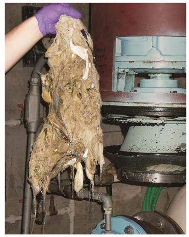
This is what happens when you flush "Disposable" or "Flushable" cleaning products. Don't be mislead by the confusing and false labels.
