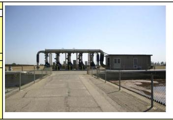
**7. Justification & Useful Life:** The District replaced blowers 3 & 4 with Neuros high speed turbo blowers completed in June 2010. The remaining blowers will be replaced with the high speed turbo blowers. Blowers 1 & 2 were placed into service in 1995 and are due for replacement.
