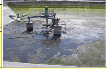
7. Justification & Useful Life: Replace4 floating aerators in Aerobic Digesters 3 and 4 with new aerator with new technology and use the aerators that are remove as a backup unit for aeration basin No. 2. We presently do not have any backup units.
