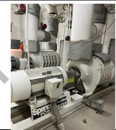
The District replaced blowers 3 & 4 with Neuros high speed turbo blowers completed in June 2010. The remaining blowers 7. Justification & Useful Life: will be replaced with the high speed turbo blowers. Blowers 1 & 2 were placed into service in 1995 and are due for replacement.
