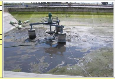
**7. Justification & Useful Life:** Replace4 floating aerators in Aerobic Digesters 3 and 4 with new aerator with new technology and use the aerators that are remove as a backup unit for aeration basin No. 2. We presently do not have any backup units.
