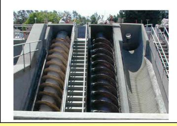
7. Justification & Useful Life: The screwlifts would be about 12 years old and will require refurbishment. The screwlifts are located in a harsh environment within the facility.
